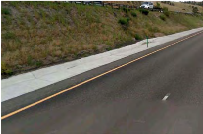
Figure 5-8 Highway Curb & Gutter (Mt. Vernon Canyon)
