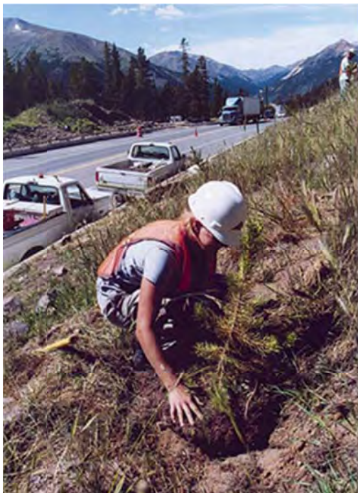
Figure 5-13 Slope Revegetation (Source: CDOT)
