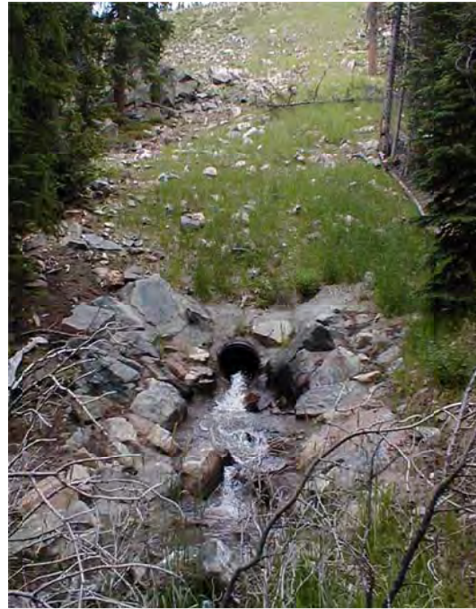
Figure 5-12 Buried Culvert Rundown with Riprap Outfall (Source: Clear Creek Consultants)
