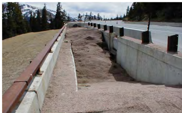
Figure 5-17 Berthoud Pass Loading Dock Sediment Traps (Source: CDOT)
