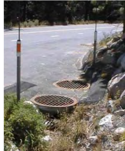
Figure 5-20 Caltrans Sand Can Sediment Tramp (Double Barrel Modified CMP) (Source: Caltrans)
