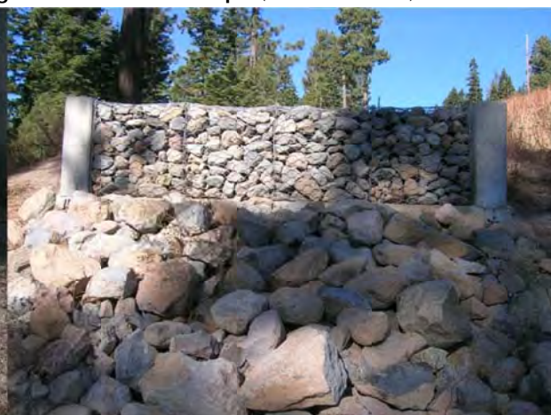
Figure 5-18 Downstream end of Caltrans Loading Dock Sediment Traps Note: Concrete bollard backstop and rock gabion (Source: Caltrans)
