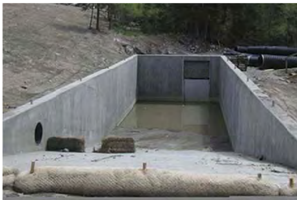
Figure 5-17 Berthoud Pass Loading Dock Sediment Traps (Source: CDOT)
