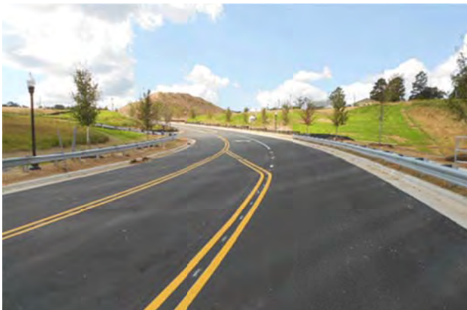
Figure 5-9 Highway Curb & Gutter - Note the Guardrails
