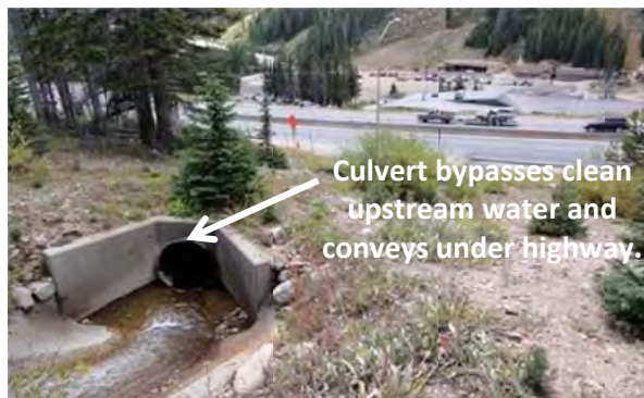
Figure 5-14 Clean Water Diversion at Loveland Ski Area Zip Creek Water Supply
