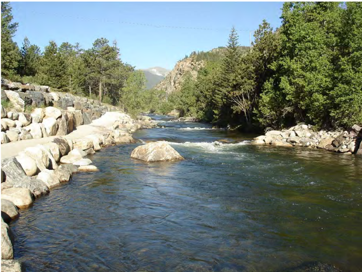
Figure 2-5 Stabilized section of Clear Creek
