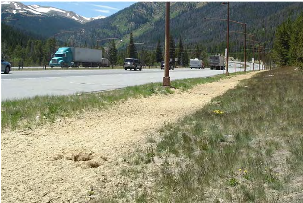
Figure 5-7 Roadside Swale
