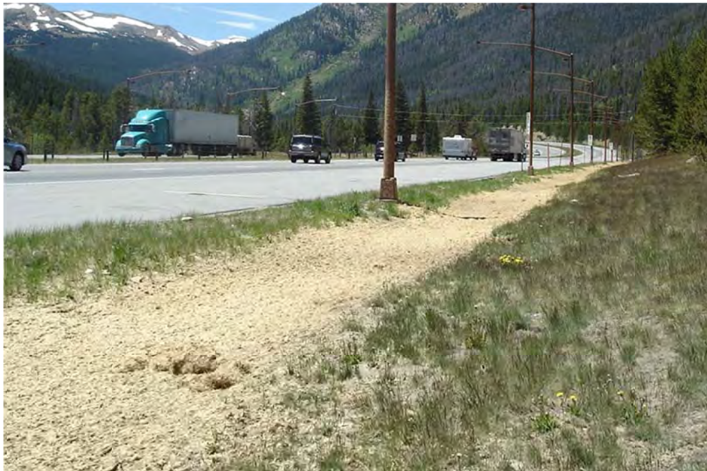
Figure 5-23 Roadside Swale
