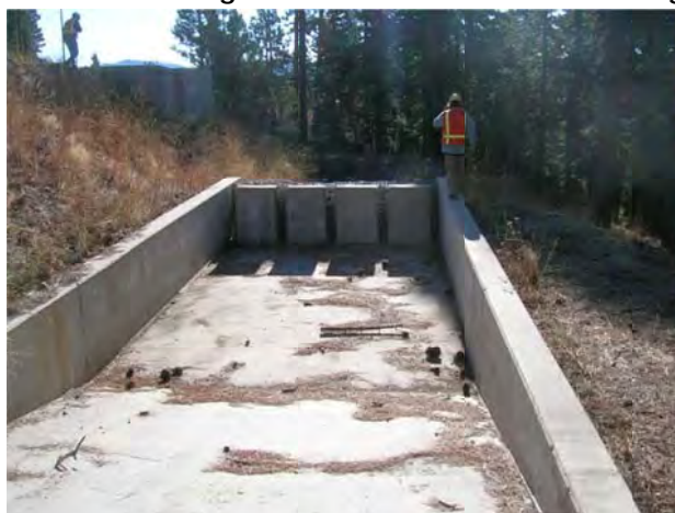
Figure 5-18 Downstream end of Caltrans Loading Dock Sediment Traps Note: Concrete bollard backstop and rock gabion (Source: Caltrans)
