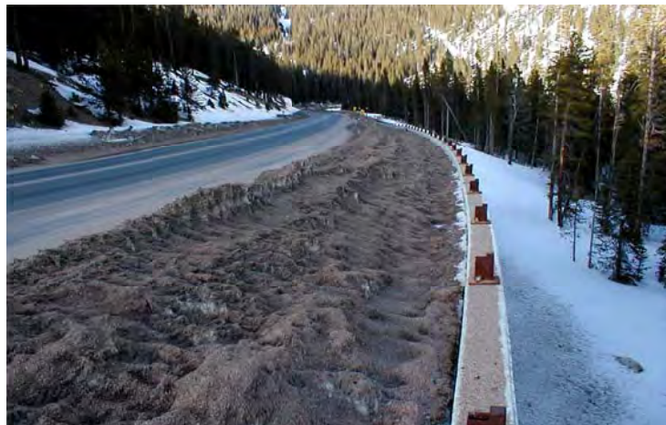
Figure 5-10 Sediment accumulation in snow storage are on Berthoud Pass (Source: CDOT)
